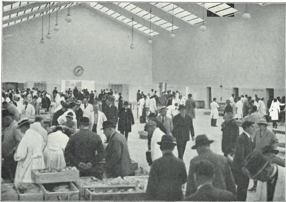
Poultry hall. (Floorage: \frac{1}{3} acre).
