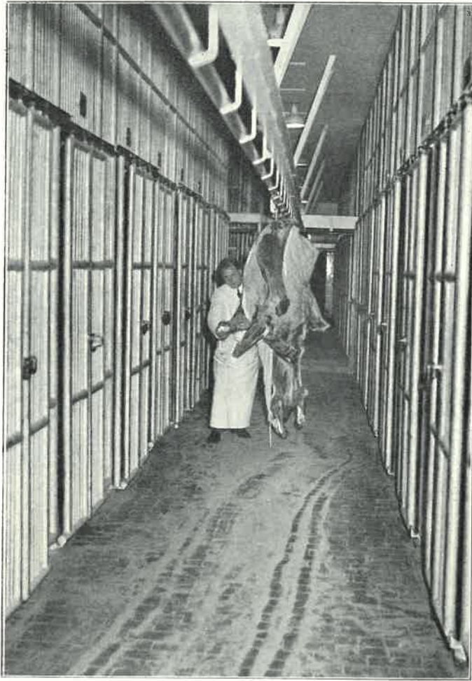
Passage between the cells of the cold store. (Floorage: 7200 square feet; number of cells: 100).
