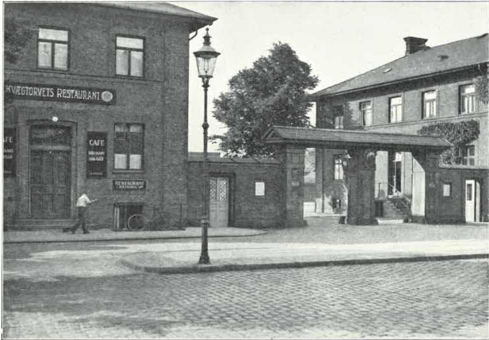
Main entrance to the cattle market. (On the right hand: the management building).
